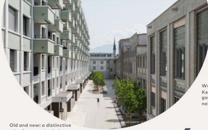
Old and new: a distinctive mix of new and existing buildings
